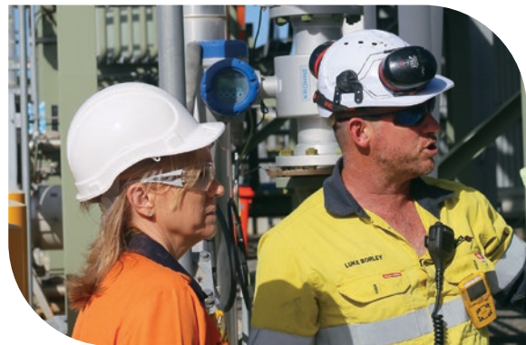
Orbost Gas Processing Plant
